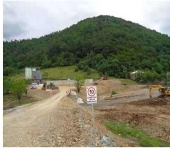
Photo 18: Muddy floor – Mud is carried by the vehicle tires to E60 road.
