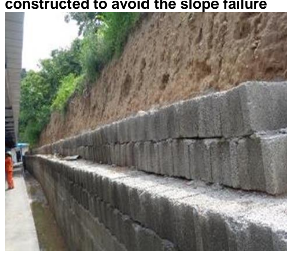
Photo 20: Retaining wall being constructed to avoid the slope failure
