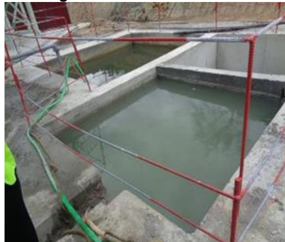
Photo14:Concrete washout recycling facility for Concrete mixer trucks at Batching Plant 1
