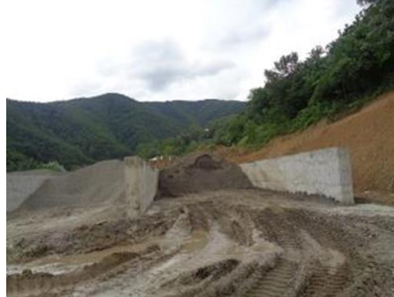
Photo 20: Retaining wall being constructed to avoid the slope failure
