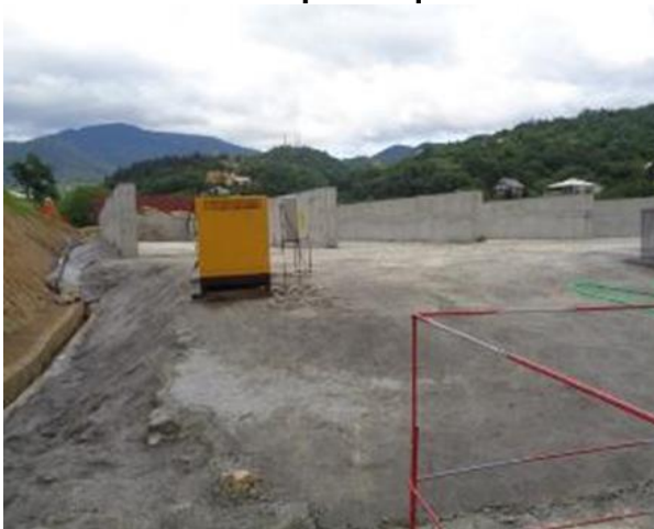
Photo13:Hard floor for material yard with storm water drains- need to be covered - storm water interceptor required
